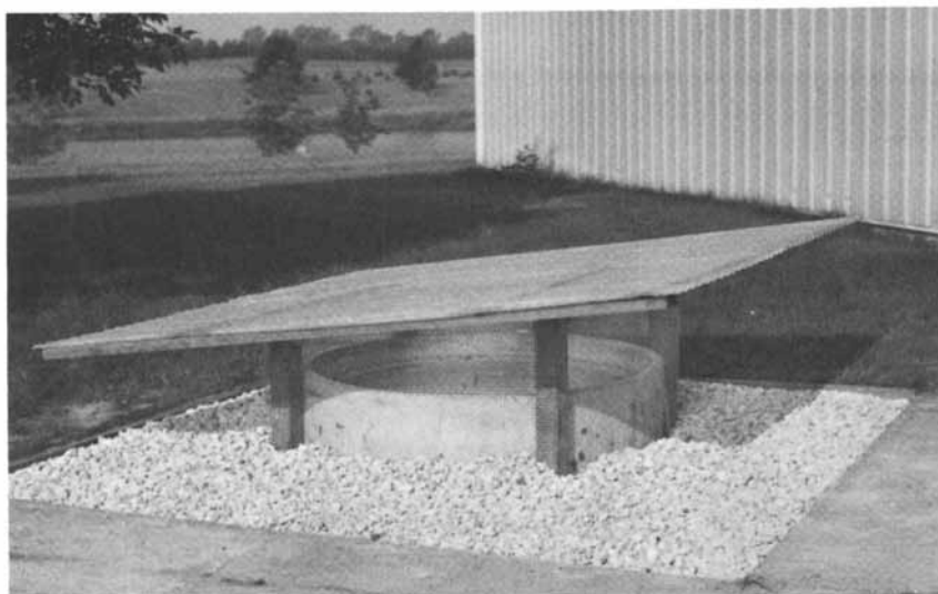
Figure 5. The above concrete unit as installed at the I.S.U. Horticulture Station as a small quantity disposal unit.
