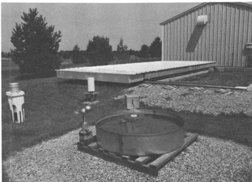
Figure 1. The concrete disposal pit with automated mobile cover and adjacent pesticide storage facility.
